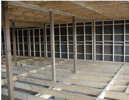
Douglas fir columns and softwood framing showing cross studding to increase insulation thickness
