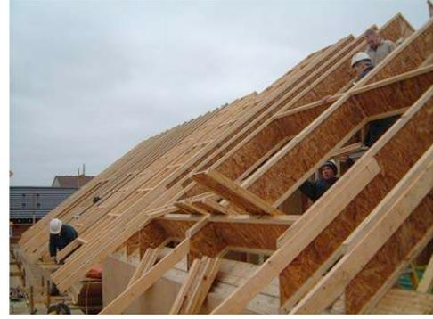
I Joists for walls and roof
